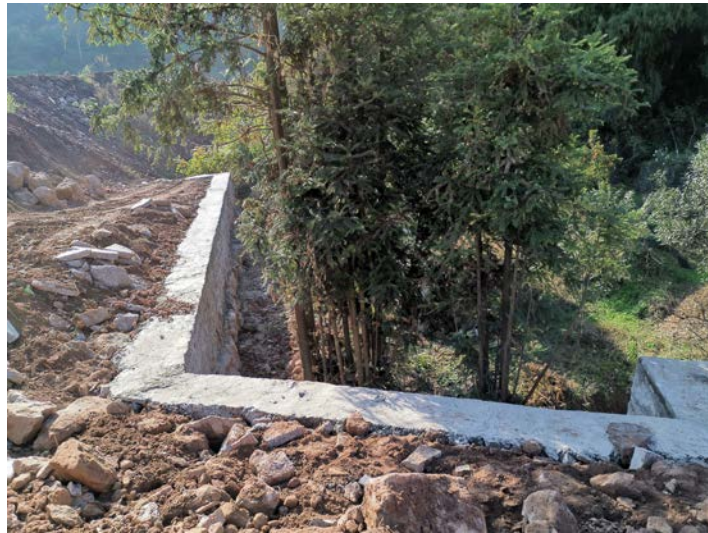
弃渣场区浆砌石挡墙
